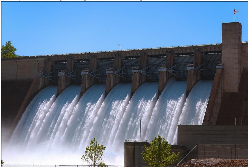
Kainji Dam (Hydro-electric Power)
