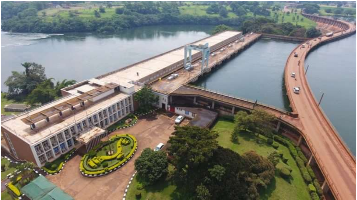
Nalubale power station
